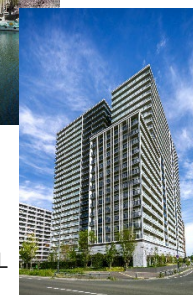
ONE PARK RESIDENTIAL TOWERS
